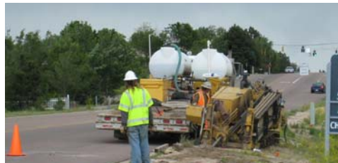
Installing the fiber-optic INET under city roads
