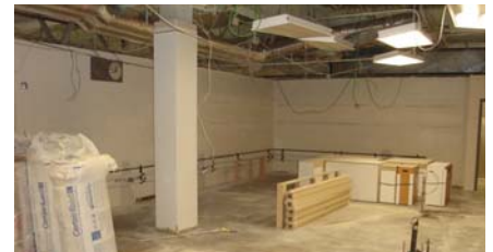
Coronado HS science room renovations
