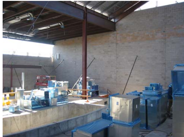
Looking over the Orchestra Pit toward the stage and south wall. Note ductwork being installed.
