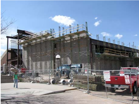
Structural elements (steel and masonry) are nearly complete.
